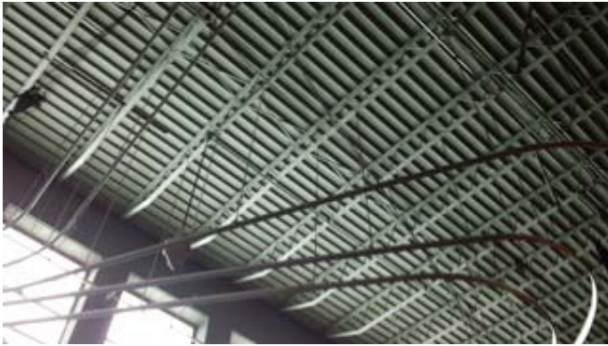
Metal Roof Deck over Stage
