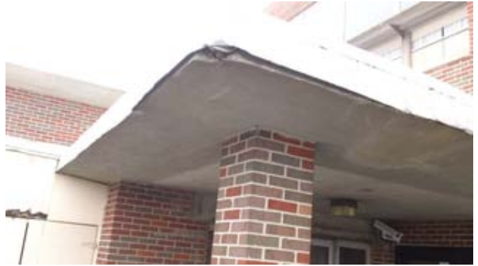
Concrete Overhang at North Entry
