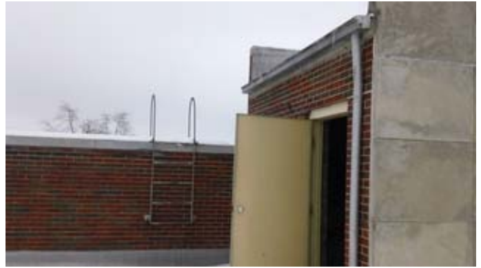
Roof Access Door
