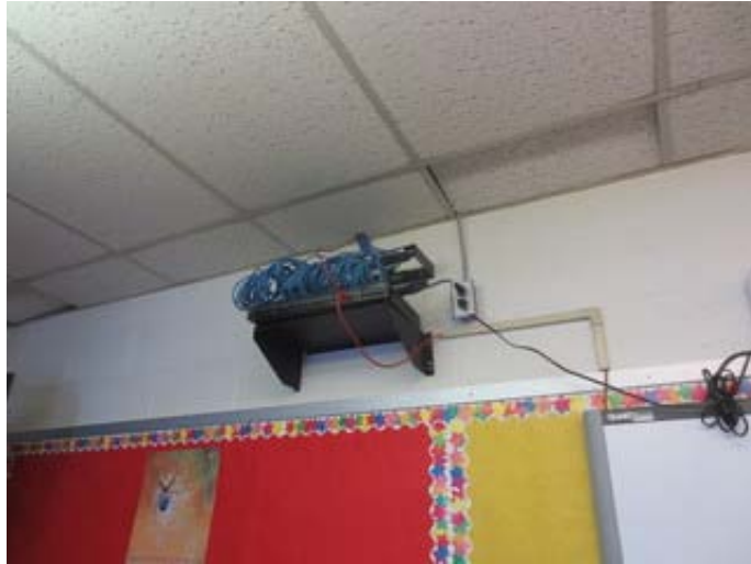
Computer Lab Data Switch
