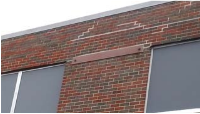
1951 Original Construction Classroom Wing Wall Bracing
