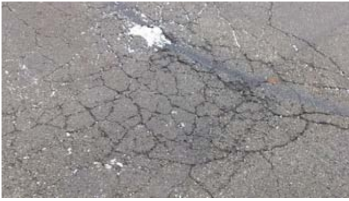
Cracking Asphalt
