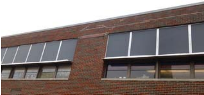
1951 Original Construction Windows
