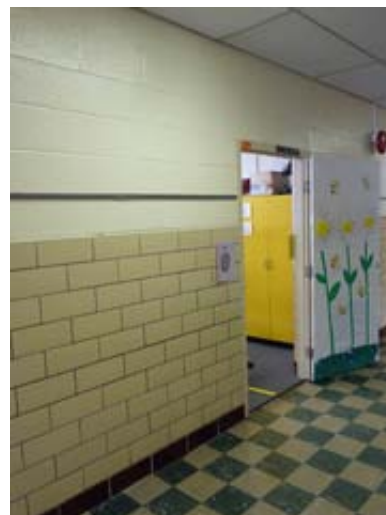
Interior Corridor Walls
