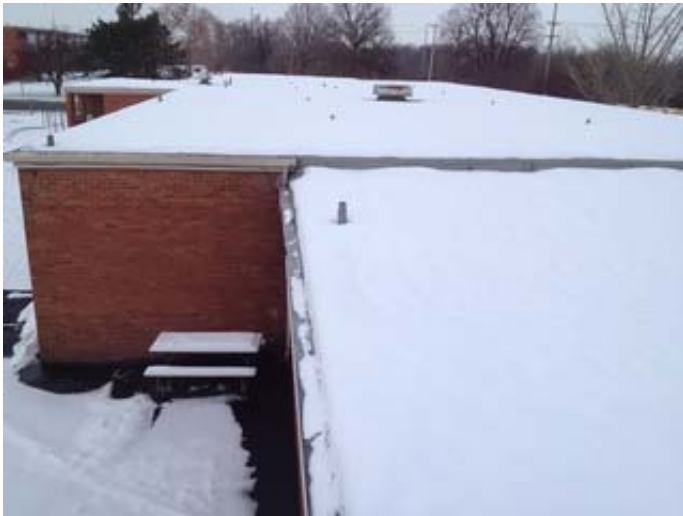
Typical Roof Condition
