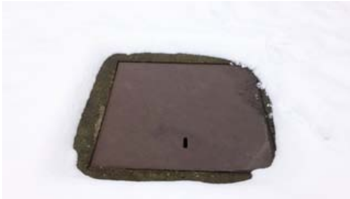
Exterior Sanitary Access
