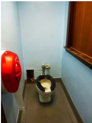
Existing Non-ADA Floor Mounted Toilet
