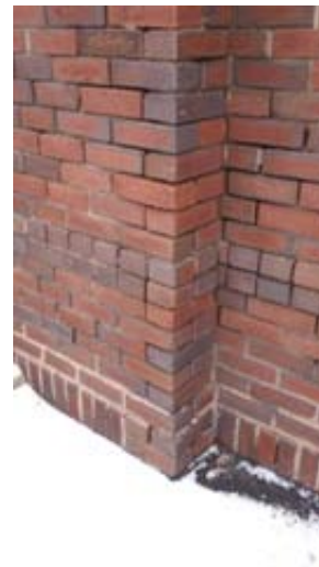
Exterior Brick Wall
