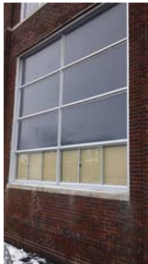
Rear Exterior Window
