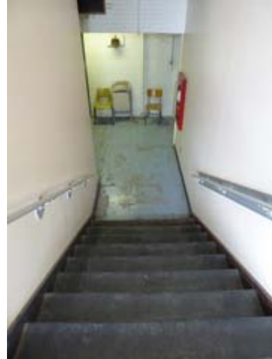
Concrete Stair and Lower Floor
