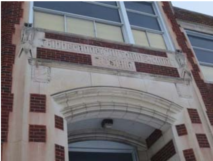
Exterior Entry Lighting
