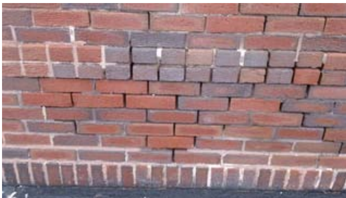
Exterior Brick Wall
