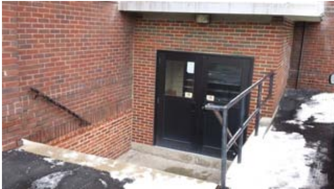
Rear Exterior Door
