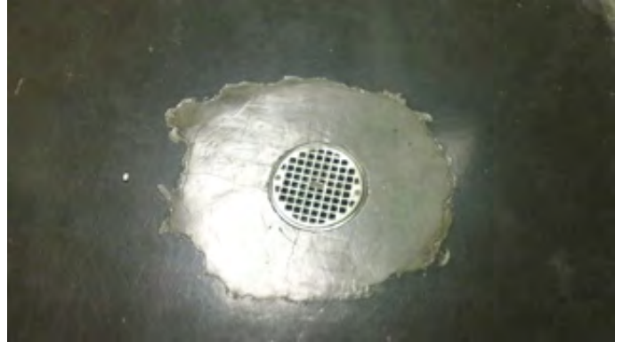
Repaired Locker Room Floor Drain
