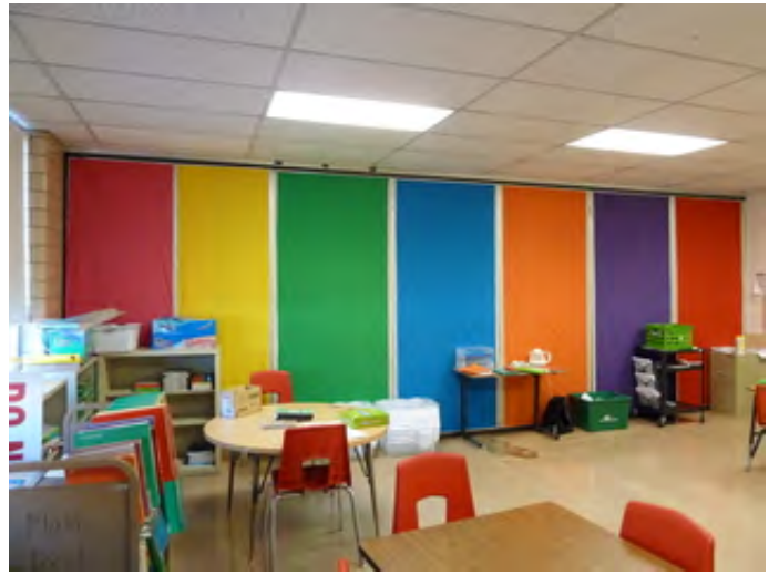
Typical Classroom Fluorescent Lighting
