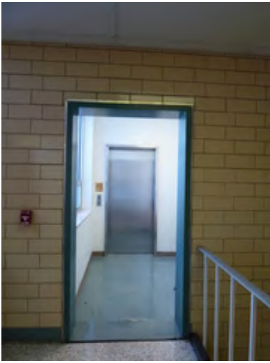
Second Level Elevator Landing
