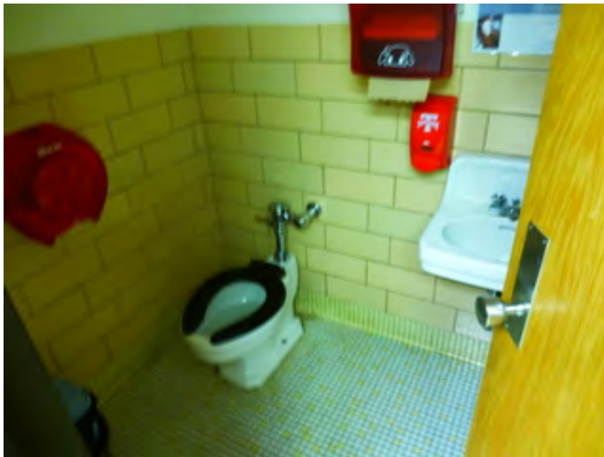
Existing Floor Mounted Toilet and Wall Mounted Lavatory
