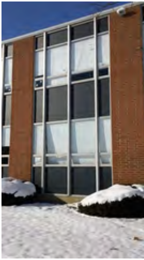
Typical Original Construction Two-Story Window System
