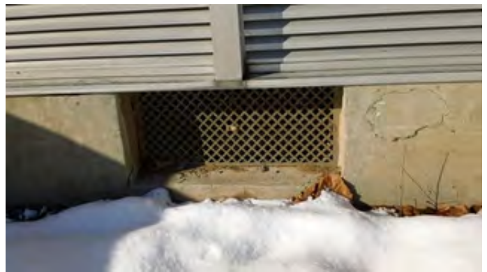
Foundation Condition at an Opening
