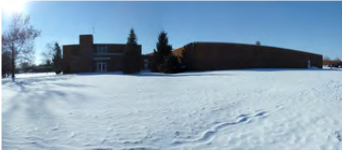
North elevation photo:
