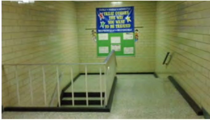
Typical Stairwell Railing System
