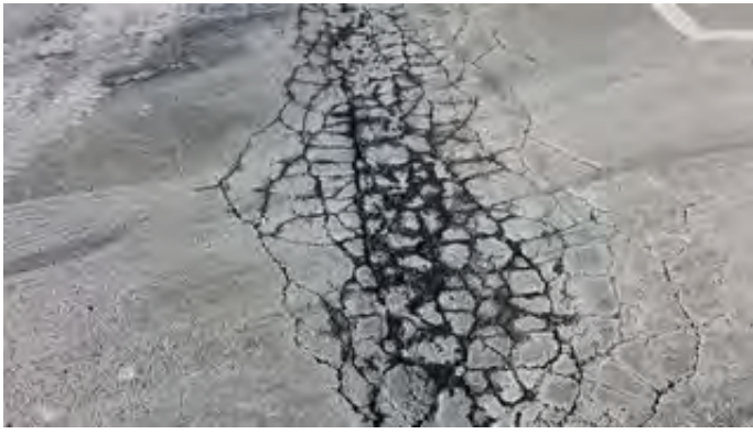
Condition of Asphalt Paving
