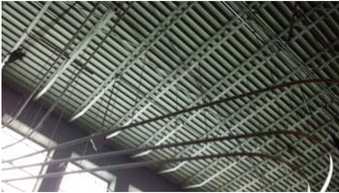
Metal Roof Deck over Stage
