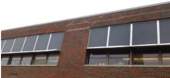
1951 Original Construction Windows
