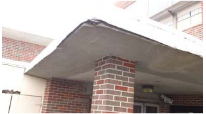
Concrete Overhang at North Entry
