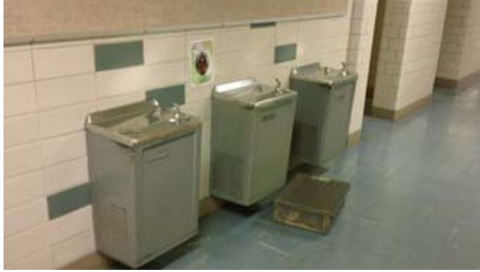
Existing Water Fountains
