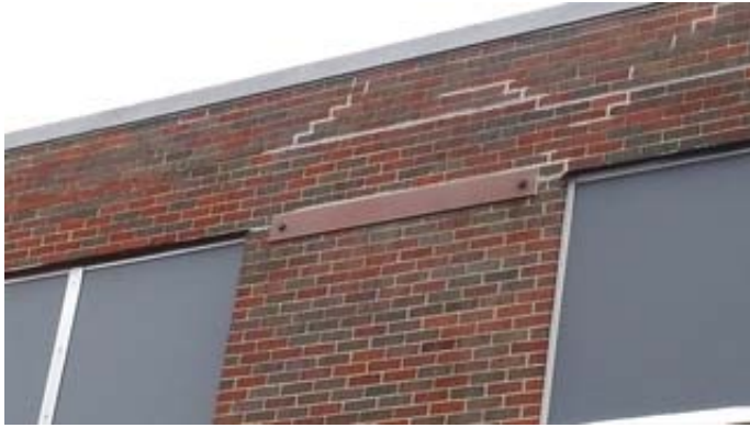
1951 Original Construction Classroom Wing Wall Bracing
