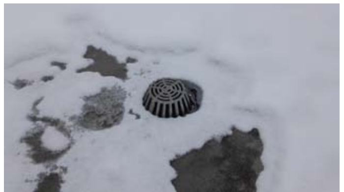
Typical Roof Drain
