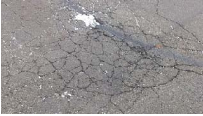
Cracking Asphalt
