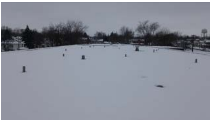
1951 Original Construction Roof
