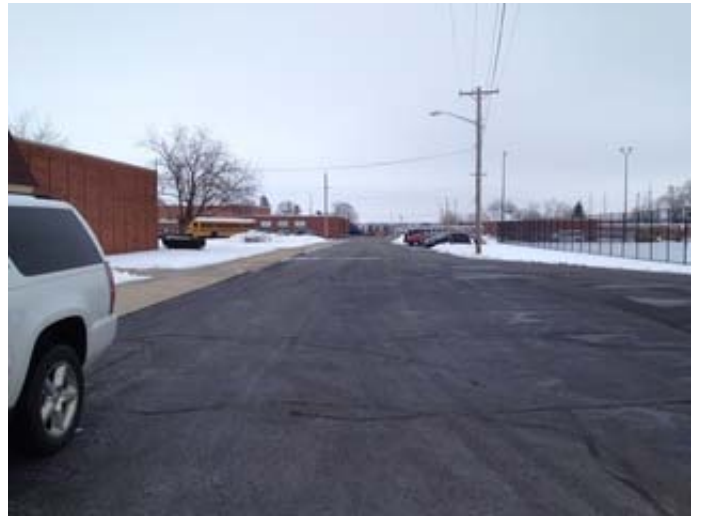
Typical Asphalt Condition
