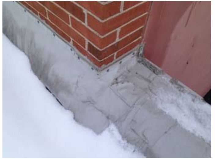
Membrane Roof Condition
