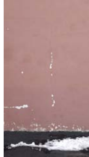
West Gym Wall Cement Plaster
