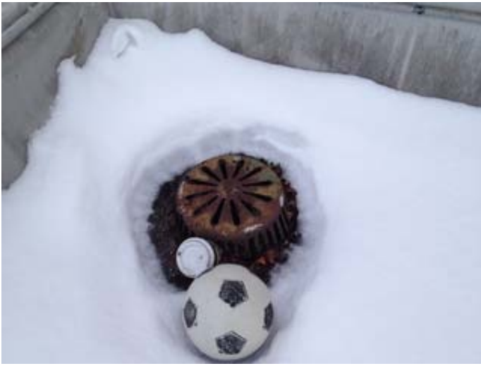
Typical Roof Vent Condition
