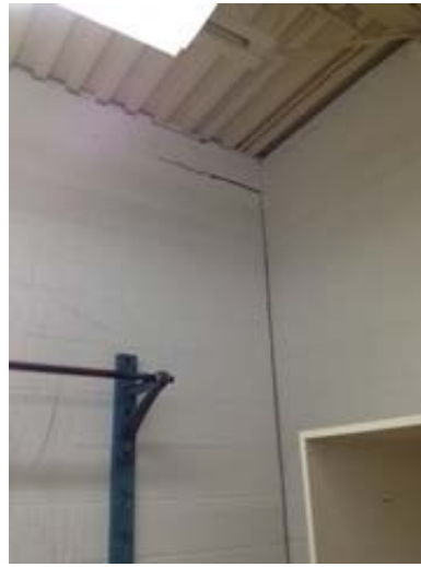
East Wall of the Multipurpose Room
