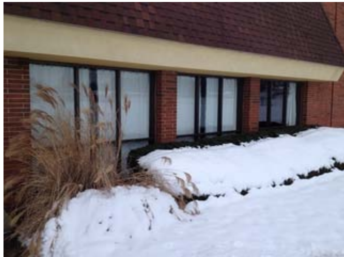
Art Room Casement Windows with Surface-Mounted Curtains
