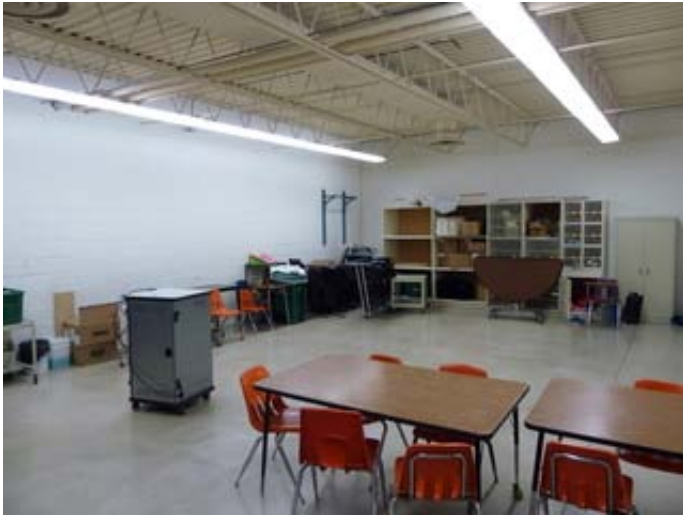
Metal Roof Deck on Open Web Steel Joists
