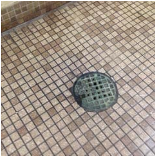
Bathroom Floor Drain
