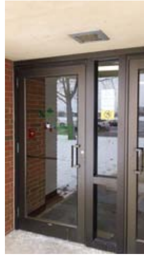
Typical Entrance Condition
