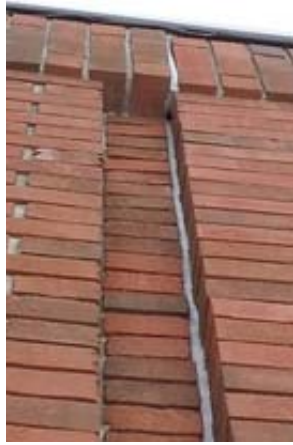
Typical Exterior Control Joint
