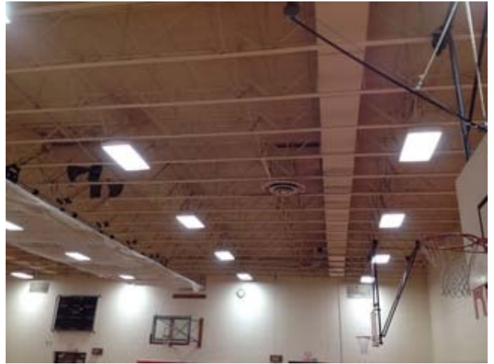
Tectum Deck on Open Web Steel Joists
