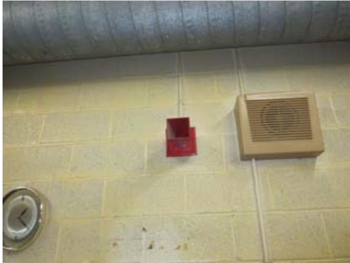
Fire Alarm Speaker and Public Address Speaker
