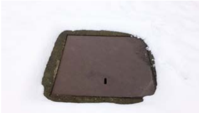
Exterior Sanitary Access
