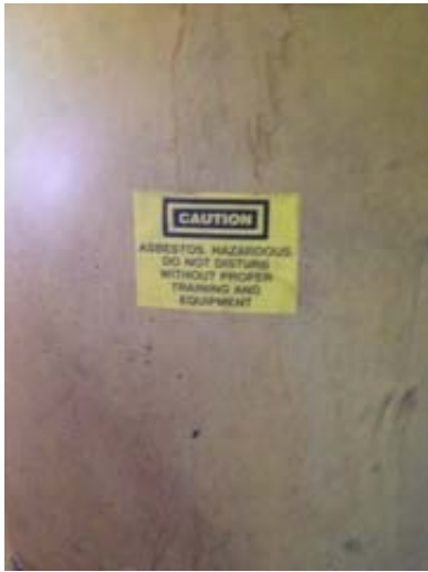
Water Tank Insulation
