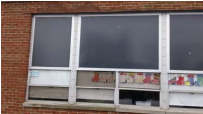
Typical Window Condition
