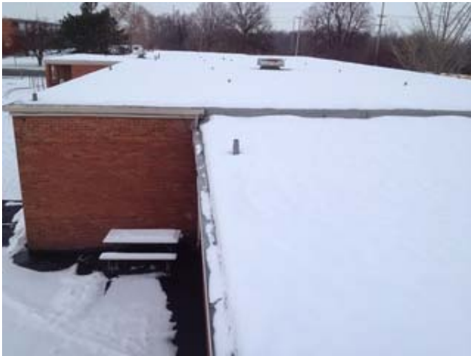
Typical Roof Condition
