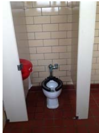
Typical Toilet Stall
