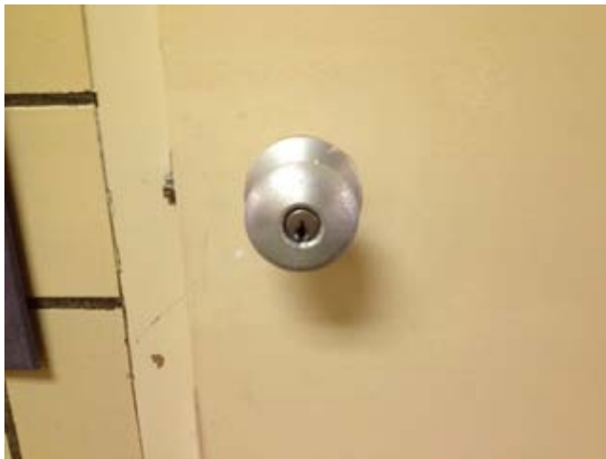
Typical Classroom Door Handle
