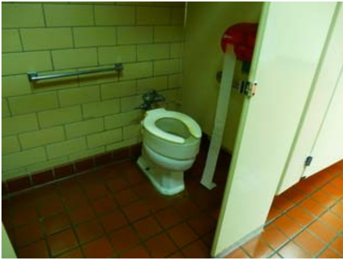
Typical Floor Mounted Water Closet
