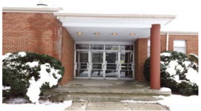
Main Entry Doors
