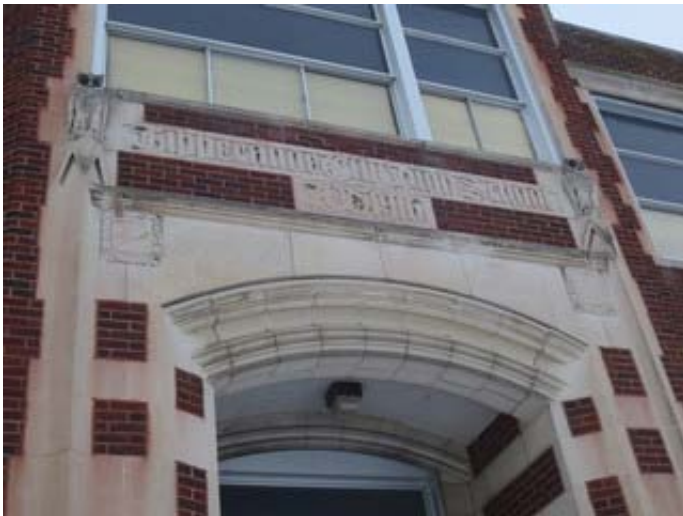
Exterior Entry Lighting
