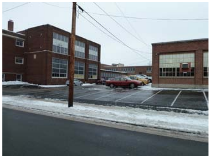
Current Parking Area
