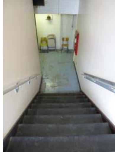
Concrete Stair and Lower Floor
