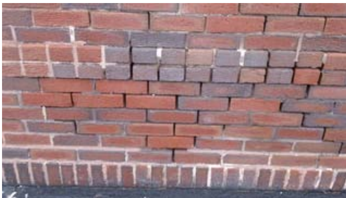
Exterior Brick Wall
