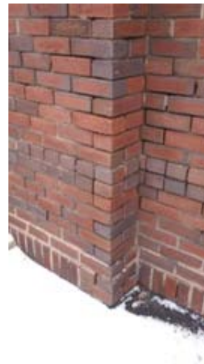
Exterior Brick Wall
