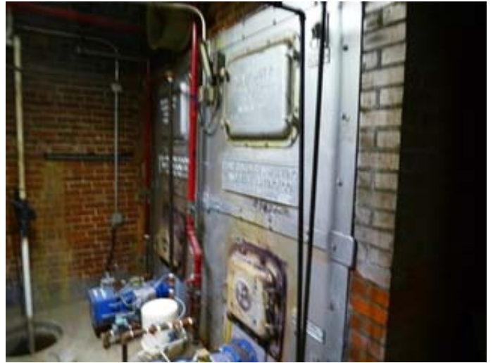
Gas Fired Forced Air Unit
