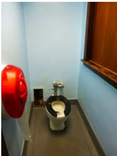
Existing Non-ADA Floor Mounted Toilet
